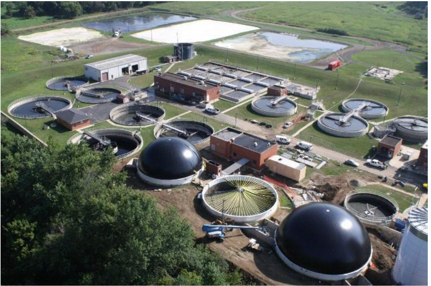
Biosolids Receiving Station and Anaerobic Digesters
