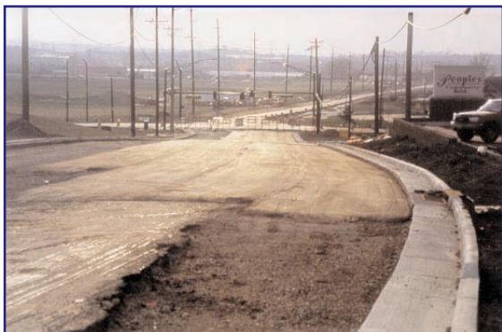
West Chester Road widening project
