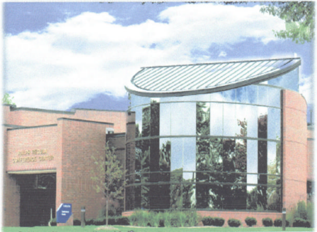
Outside view of Ralph Regula Conference Center
