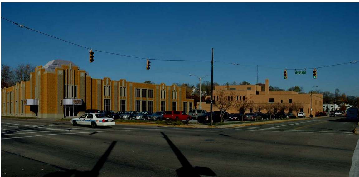
Computer generated picture of proposed police facility (left); existing City Hall (right)
