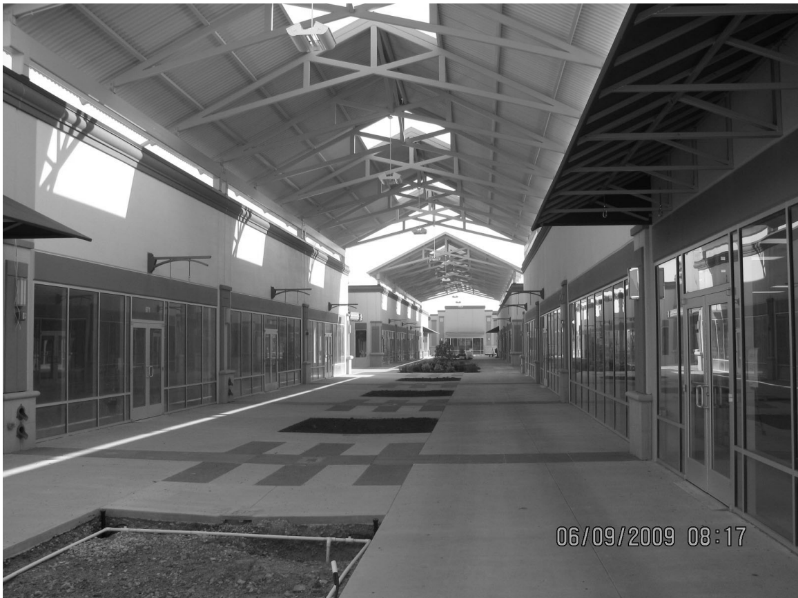
INSIDE THE CINCINNATI PREMIUM OUTLETS DEVELOPMENT UNDER CONSTRUCTION
