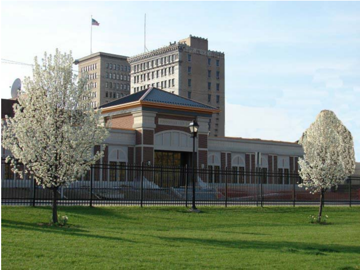
New Municipal Building
