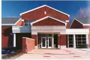
Solon Branch Project Type: Renovation Completion – May 2, 2012
