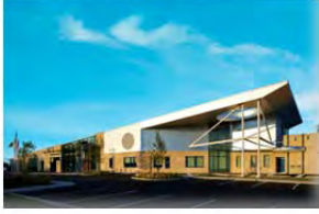
North Royalton Branch Project Type: New Construction Grand Opening – August 3, 2013
