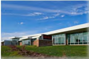
Parma Branch Project Type: New Construction Grand Opening – October 26, 2013
