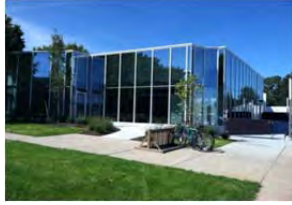
Brook Park Branch Project Type: Renovation Completion – August, 28 2014
