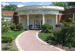
Chagrin Falls Branch Project Type: Renovation Completion – June 15, 2013
