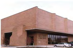
Maple Heights Branch Project Type: Renovation Completion – July 10, 2014
