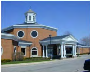
Independence Branch Project Type: Renovation Completion – Spring 2014
