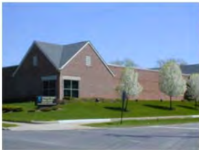
Southeast Branch Project Type: Renovation Completion – Spring 2014
