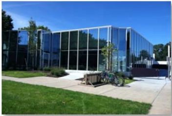
Brook Park Branch Project Type: Renovation Completion – August 28, 2014
