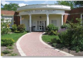
Chagrin Falls Branch Project Type: Renovation Completion – June 15, 2013
