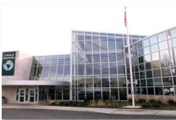
Fairview Park Branch Project Type: Renovation Completion– August 1, 2012
