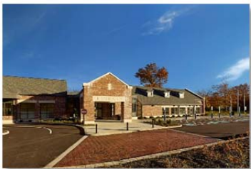
South Euclid-Lyndhurst Branch Project Type: New Construction Grand Opening – October 18, 2015
