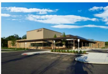
Mayfield Branch Project Type: New Construction Grand Opening – April 20, 2013
