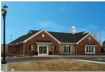
Olmsted Falls Branch Project Type: New Construction Grand Opening – February 23, 2013
