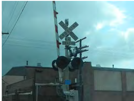
South Hamilton above grade railroad crossing
