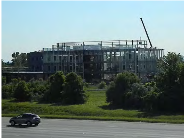
New Christ Hospital Facility near the Liberty Way Interchange
