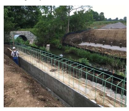
Resource Management was also critical as stream erosion of Alum Creek at Three Creeks was mitigated by construction of a stream bank.
