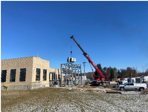
Photo 1: Construction of standby generator
