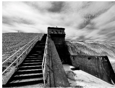
Spillway Stairs & Gate House
