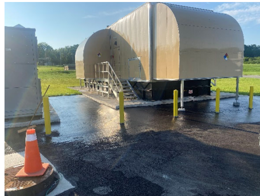
Photo 2: Generator housing installation.
