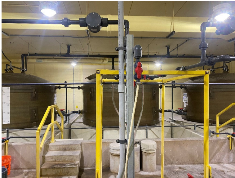
Photo 1: G-148 Fluoride System Replacement
