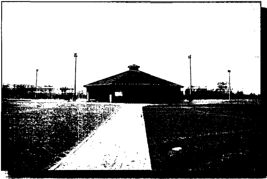
Concession Building at the new lighted baseball facility • 1997
