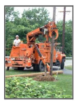
THE INSTALLATION OF ONE NEW POLE TO REPLACE TWO EXISTING POLES IS ONLY ONE OF THE MANY UPGRADES THE CITY'S ELECTRIC LINE CREWS ARE CONTINUALLY PERFORMING.
