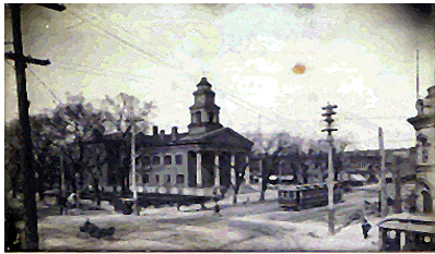
Greene County Courthouse destroyed by fire in 1900
