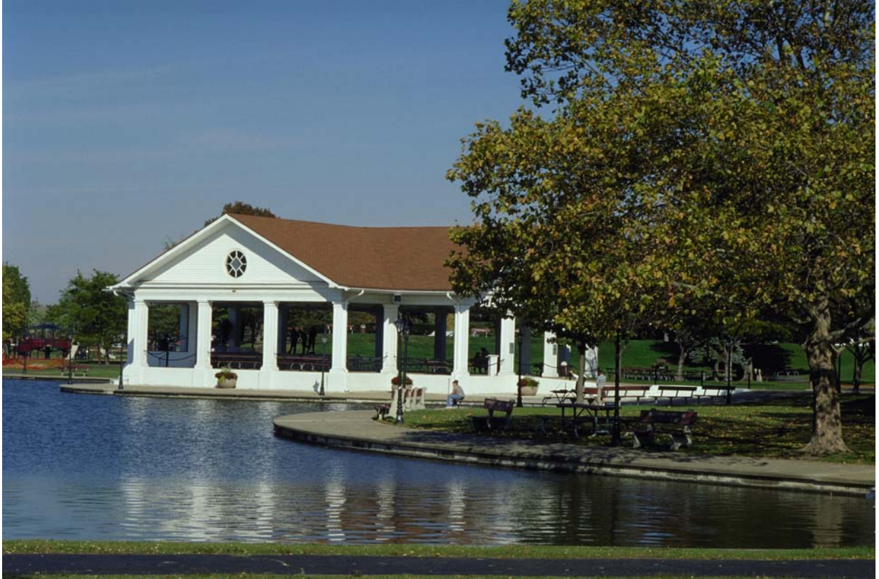
A view of the Pavilion at Shawnee Park located in downtown Xenia.
