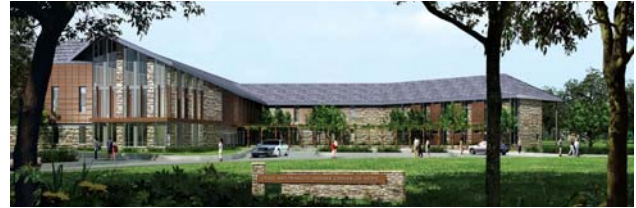
Lindner Center or HOPE, under construction in 2007, will provide state-of-the-art mental health care.
