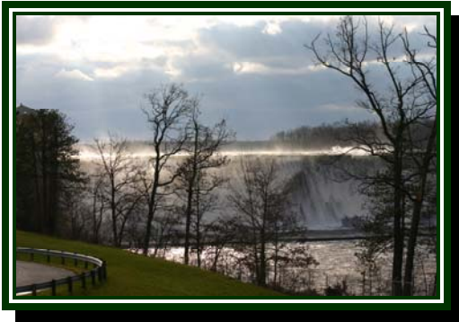
Photo No. 1 – Meander Dam
