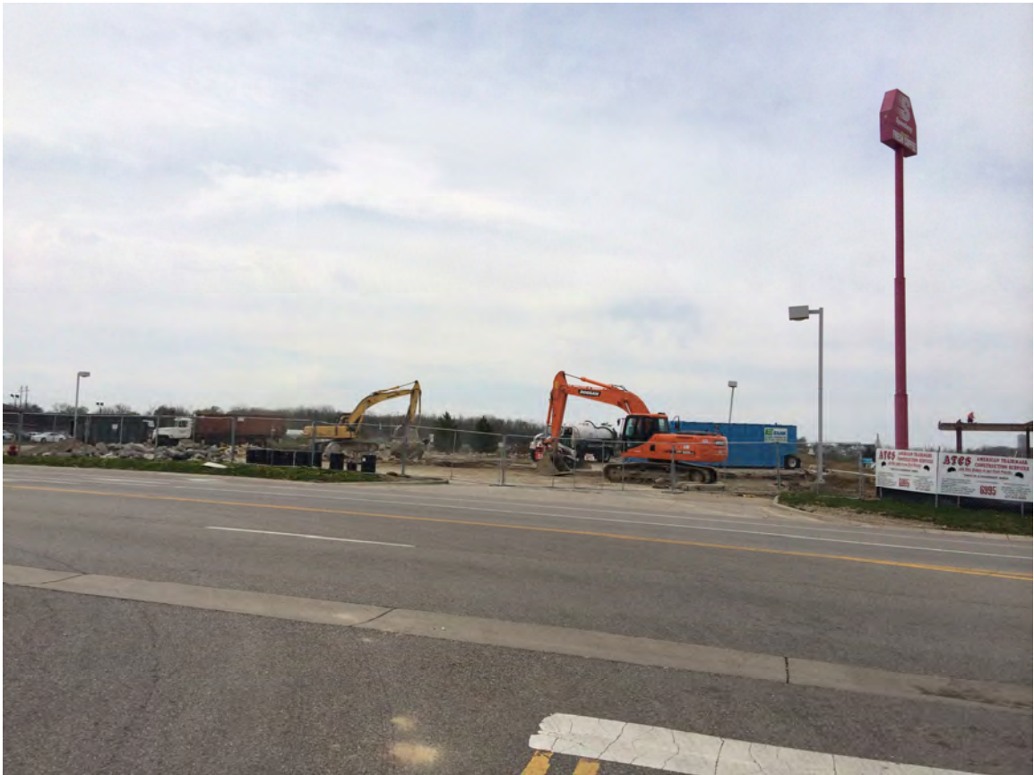
Speedway Gas Station Demolition
