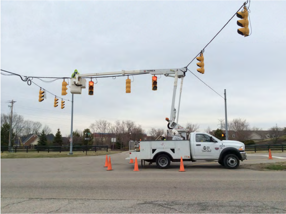
Crews Installing Cable Along State Route 63 for Fiber Lights
