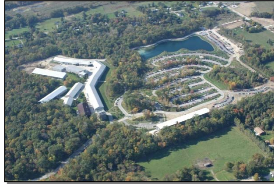
Figure 6 – Aerial View of Business Campus
