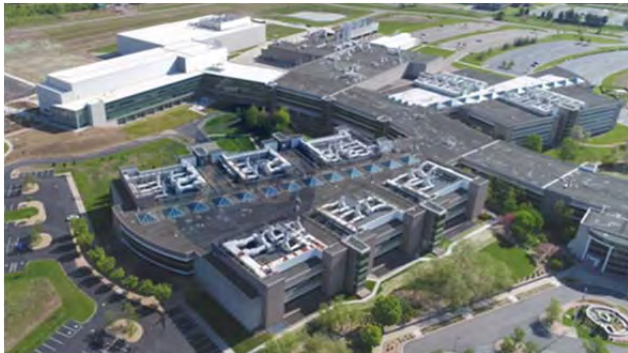
P&G Beauty Innovation Center, home to the Global Beauty and Global Health, completes its final year of construction and hosted its grand opening in May of 2019. The 241-acre campus and now 2 million square-foot facility is Mason & Warren County’s largest employer.
