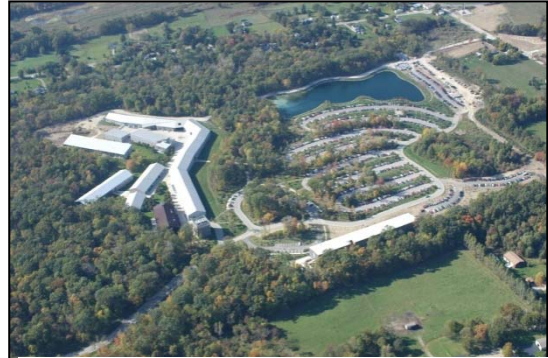
Figure 6 – Aerial View of Business Campus
