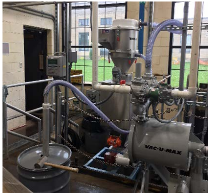
New vacuum feed Potassium Permanganate educator system
