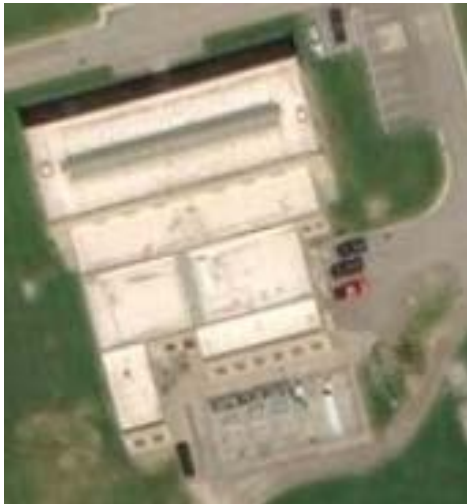
High Service Pump Station Building where the Plant Standby Power project will take place.
