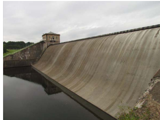
Photograph of the principal spillway.
