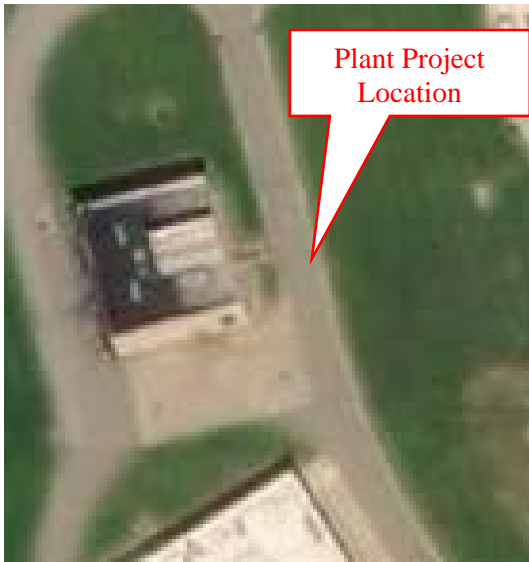
Photograph of the Carbon Building where the new carbon and potassium permanganate feed will be replaced and incorporate into the new dam embankment.
