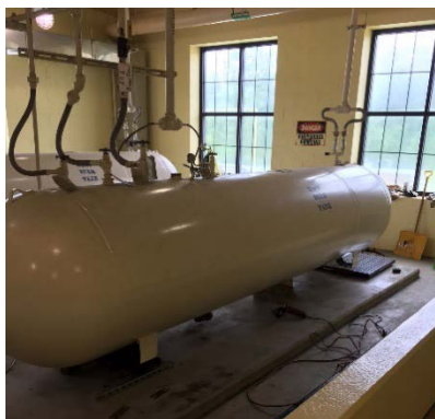
New ammonia system upgrade including new scales, piping and fittings.
