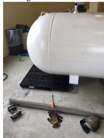
Installation of new scale on south tank.
