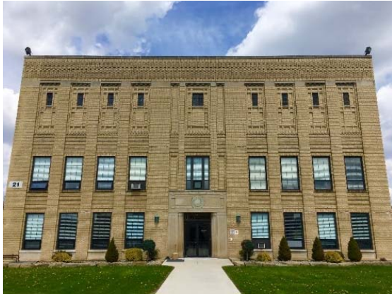
Photograph of the Administration Building (No. 21)
