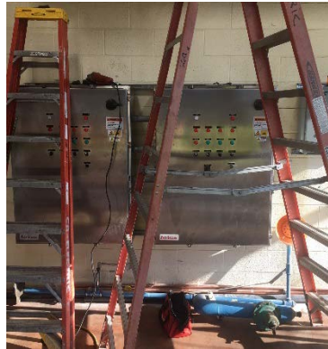
Installation of control panels for new potassium permanganate feed system.
