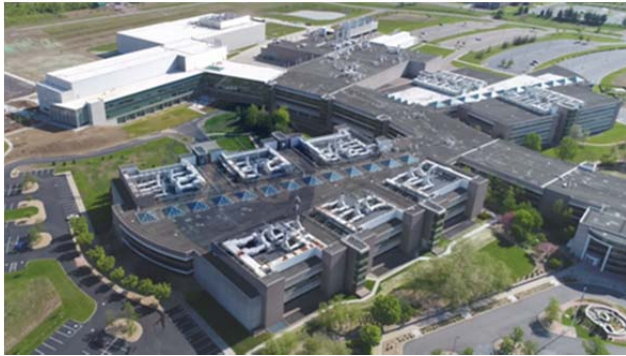
P&G Beauty Innovation Center, home to the Global Beauty and Global Health. The 241-acre campus and now 2 million square-foot facility is Mason & Warren County's largest employer.
