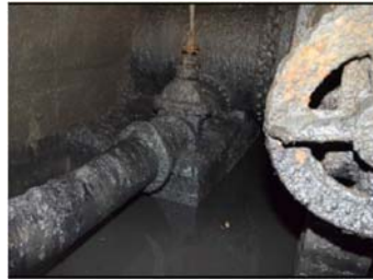
Photo 2: Existing valve proposed for replacement in the Phase IV Project.
