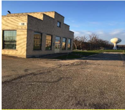
Photo 2: Photograph of the east side of the Carbon/Permanganate Building
