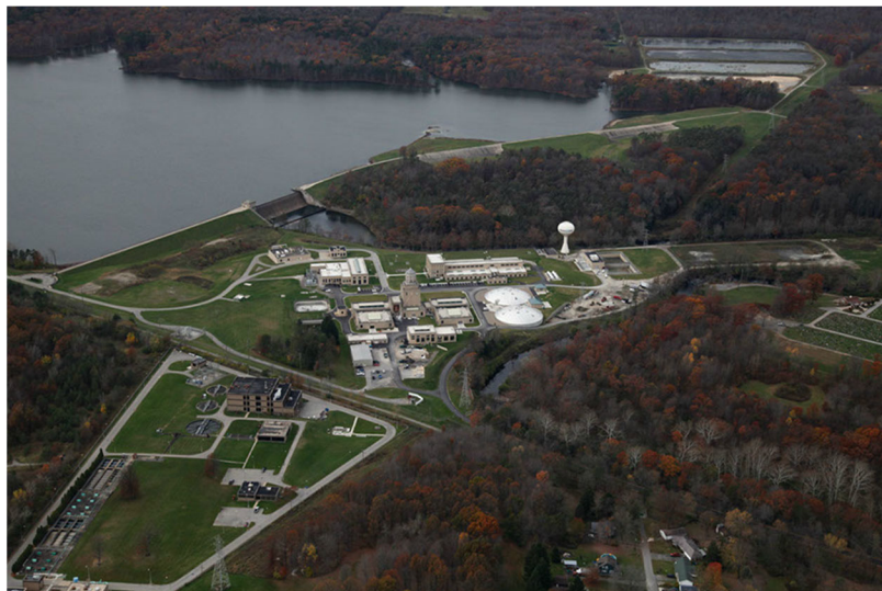
West View of MVSD
