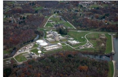
East View of MVSD
