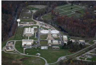
North View of MVSD
