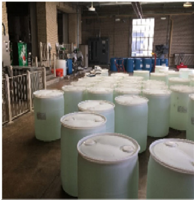
Photo 1: Existing Temporary Chemical Feed Configuration to be replaced by new bulk chemical feed system.
