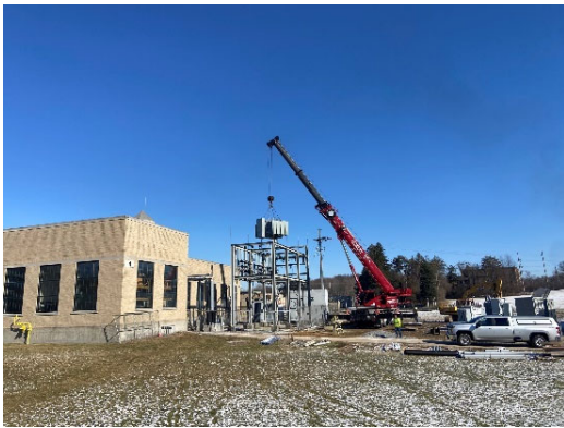
Photo 1: Construction of standby generator
