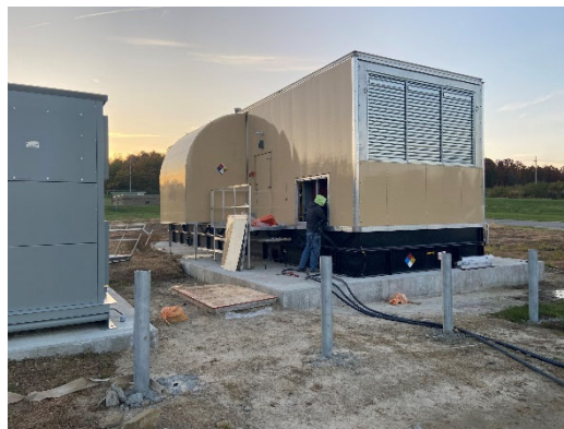
Photo 2: Generator housing installation.
