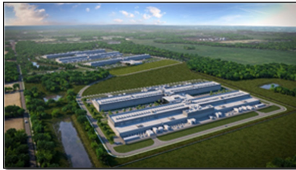
Figure 4 – Facebook New Albany Data Center
